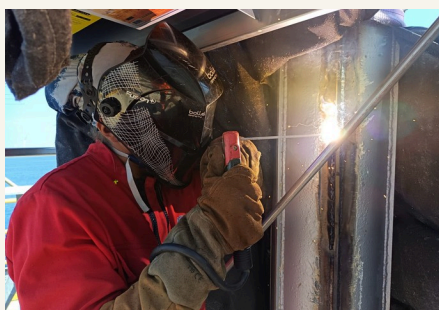
■ WELDING ON AN OFFSHORE WIND FOUNDATION
